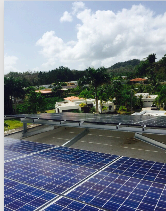
Residential PV system installed in Guaynabo and financed by JOC in 2016. This project produce 5 KWh of clean energy and, due net metering system reduce the utility bill to $3 monthly.
